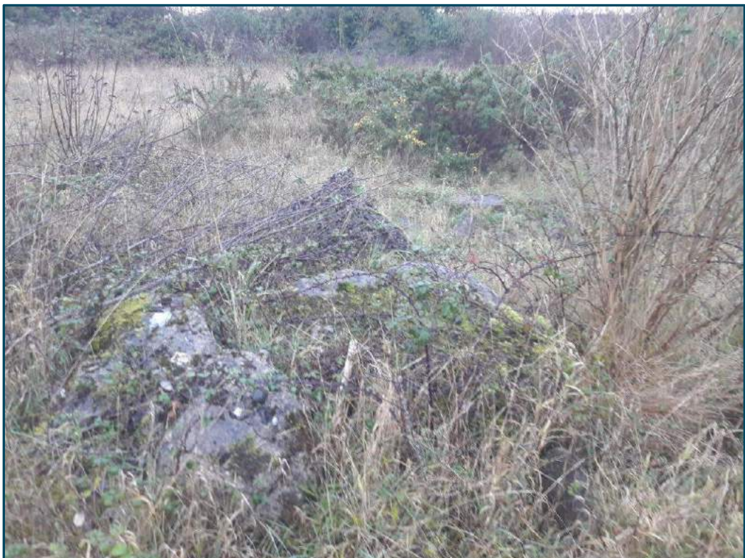
Plate 2 – Overgrown concrete debris present on site
