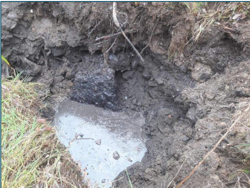
Plate 6 – Shallow groundwater accumulating in TP107
