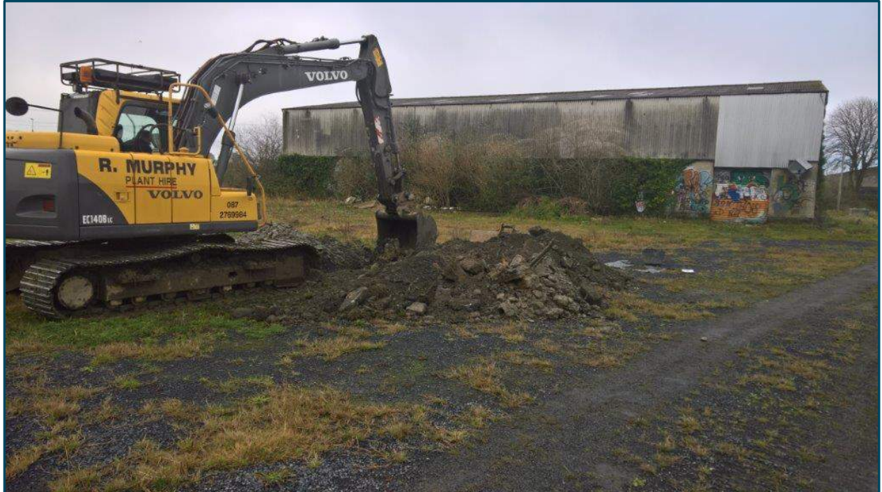
Plate 7 – Excavation of TP115
