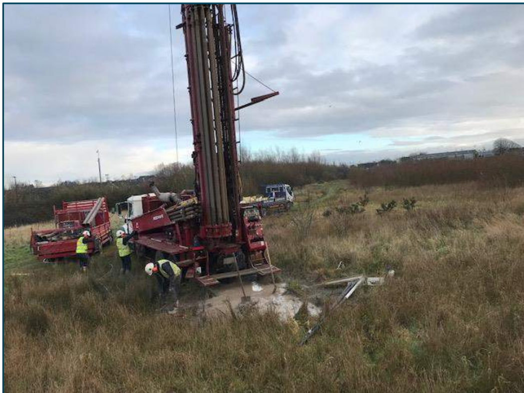
Plate 8 – Dilling works at MW-101 location
